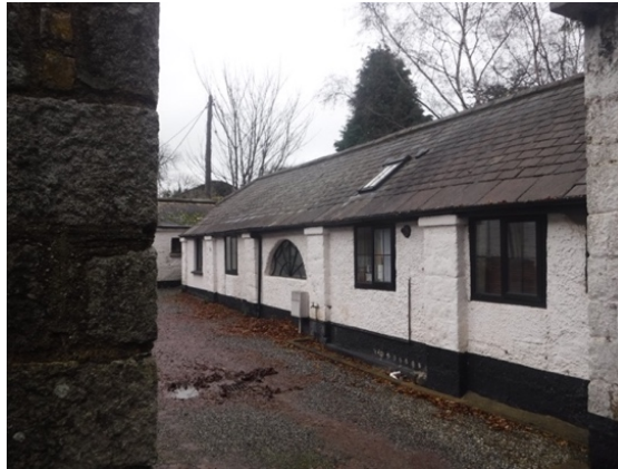
Figure 18.43: Outbuildings to Corke Lodge.
